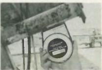
AN "INCLINOMETER" is a valuable tool in TVRO installation. Here we see how one commonly available unit is used.
